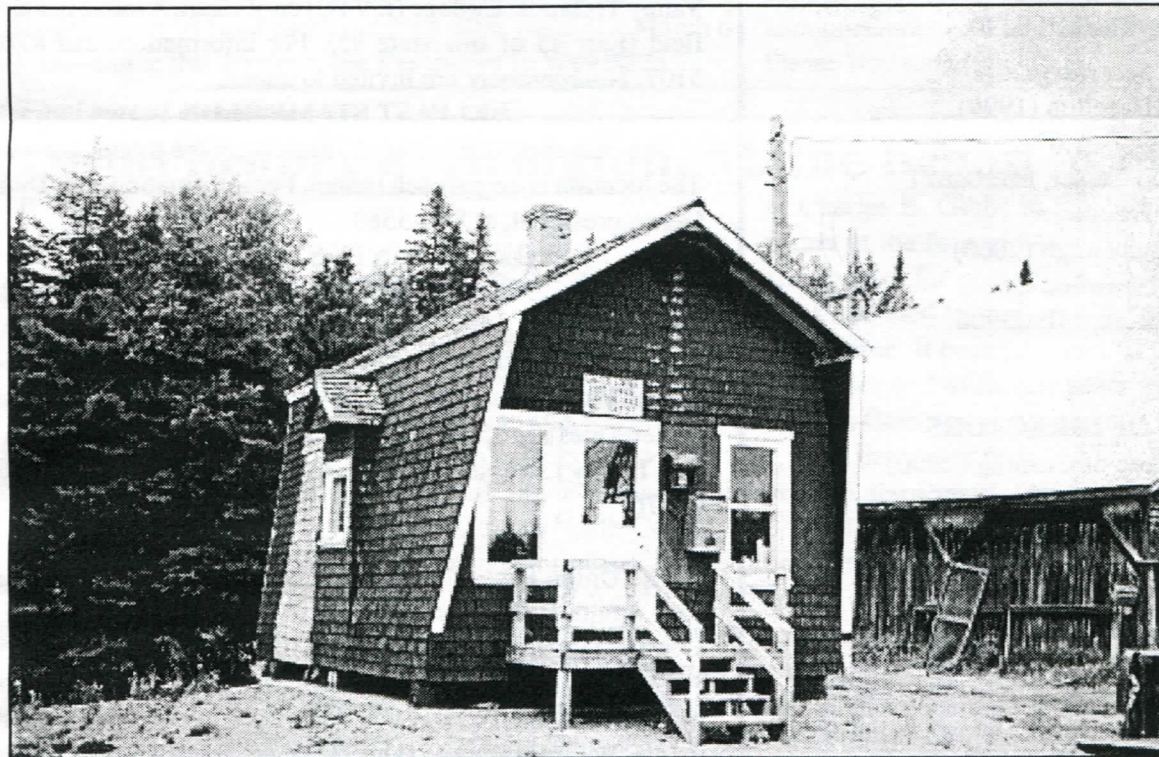
The post office at Clayton Lake, the most remote in all New England
