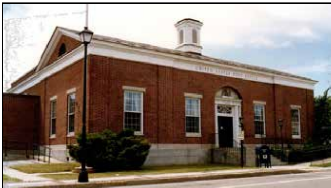
The post office in South Portland, Maine.
